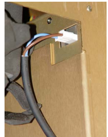
Chiller Power Wire Harness Figure 7.9
