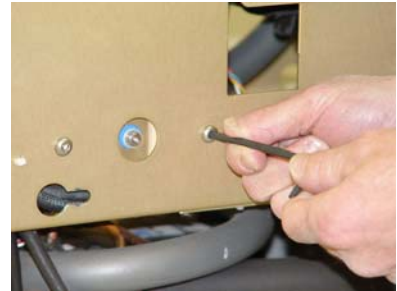
Circulating Pump Mounting Screws Figure 7.20
